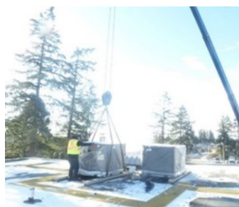
Birch building ACCU replacement units. Birch building new cooling coils installation complete.
